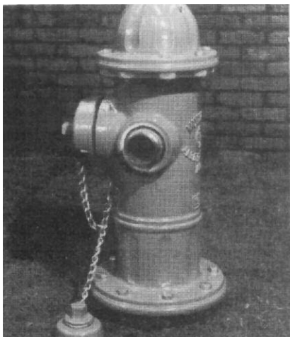
2. Remove stainless steel Nozzle Lock by driving it out with a pointed tool and hammer.
