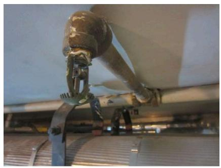
Because this fire sprinkler points down, the spur-shaped deflector should be convex rather than concave. That's a tell-tale sign that this is an upright fire sprinkler—which isn't listed for this use. Image source: *Fire Protection Deficiencies*
